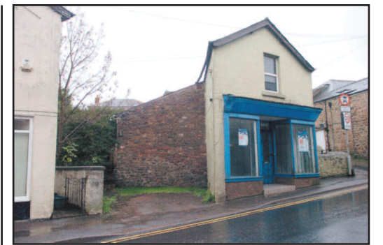
THE High Street in Cinderford where a water leak remains unresolved.
